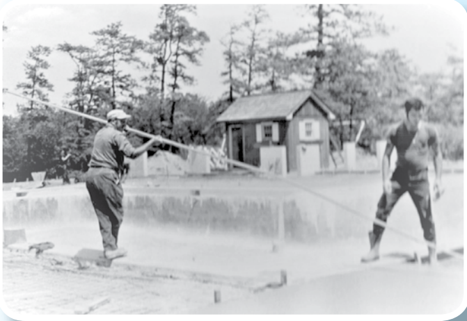
Building Willow Pool
